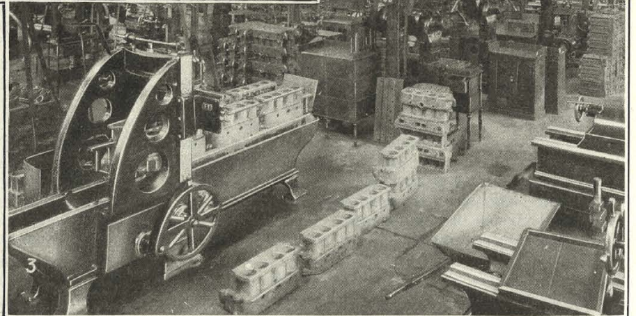
Fig. 3—Straight-line cylinders being planed on their mating surfaces. This method is in marked contrast to that employed in plants where the production is large
